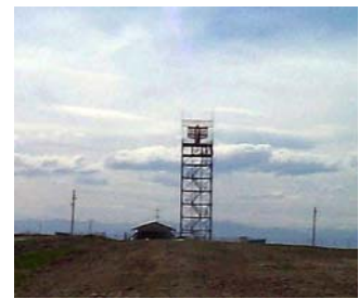
FAA Airport Surveillance Radar
