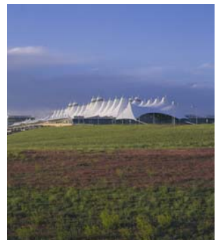
DEN's Terminal tent roof view from the South.
