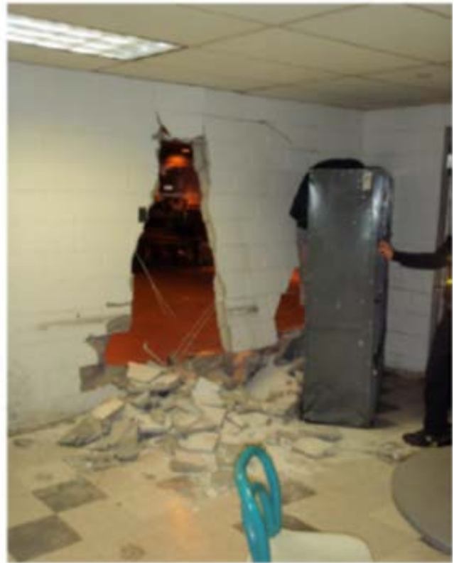
Figure 8-1: Concourse B: Tug Damage to Wall
