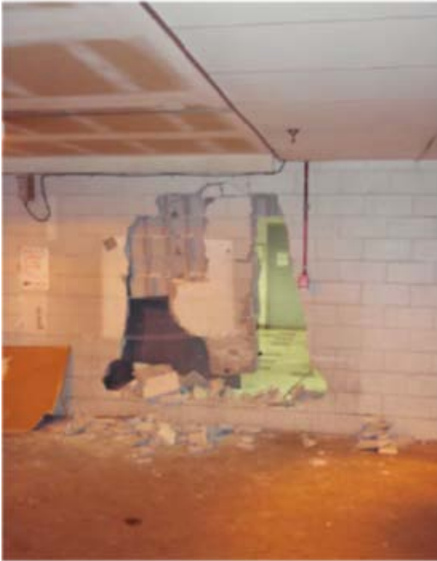
Figure 8-1: Concourse B: Tug Damage to Wall
